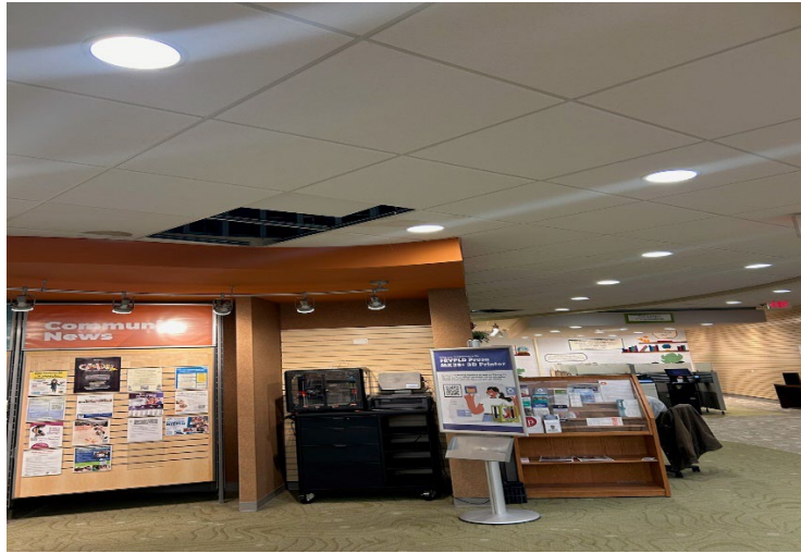
Ceiling area damaged by leak
