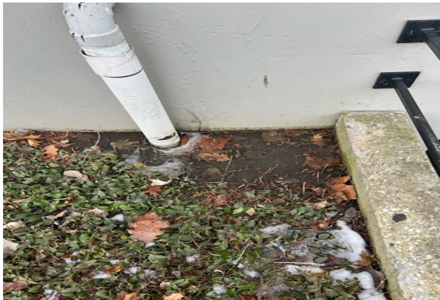
Potential source of leak
