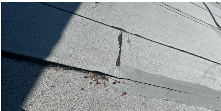
Spilt seams identified by DCG Roofing
