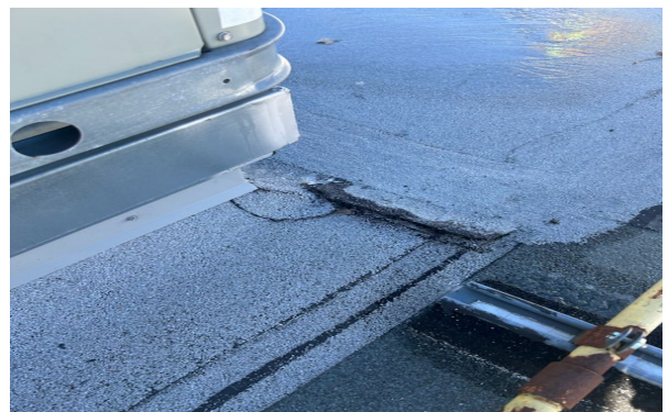
Spilt seams identified by DCG Roofing
